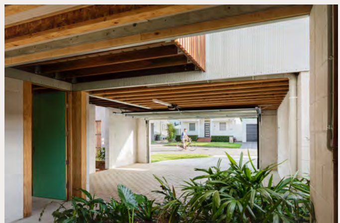
↑ Below the flood level, materials are water-resistant and the space has been kept open to the back yard to allow any floodwaters to move through unimpeded.
